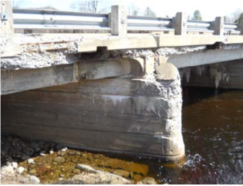
Deteriorated deck & pier
