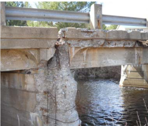
Deteriorating Pier and Deck
